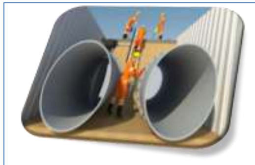
Figure 9: Twin 1.6m diameter Pipelines
