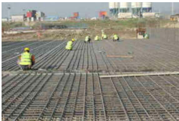
WTP: Reinforcement of W40 Slab- Block B2
