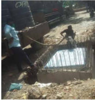
Curing the walls of DMA chamber
