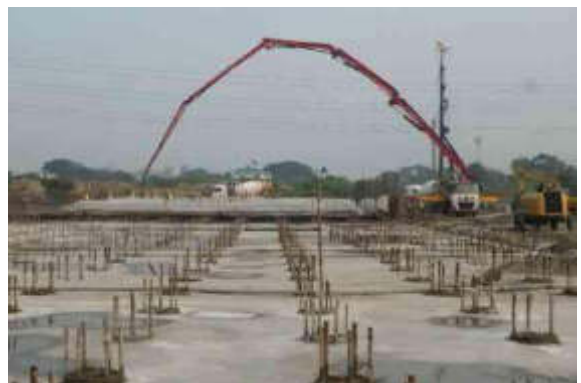
WTP: Concrete pouring at Block B1 of W40
