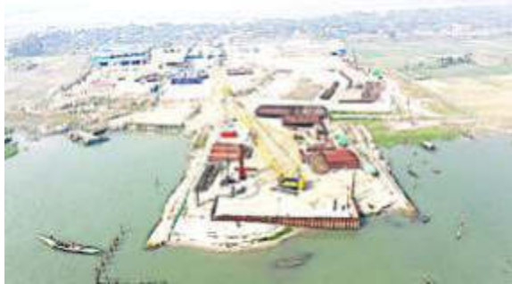
Intake: Progress in sheet piling
