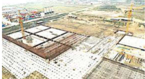
WTP: Reservoir work in progress
