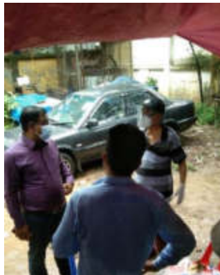
CM in visit to see pre commissioning on 29.07.20 at DMA 616 segment -3
