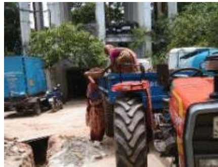
Removing excavated earth by women laborer from DWASA System compound DMA 614
