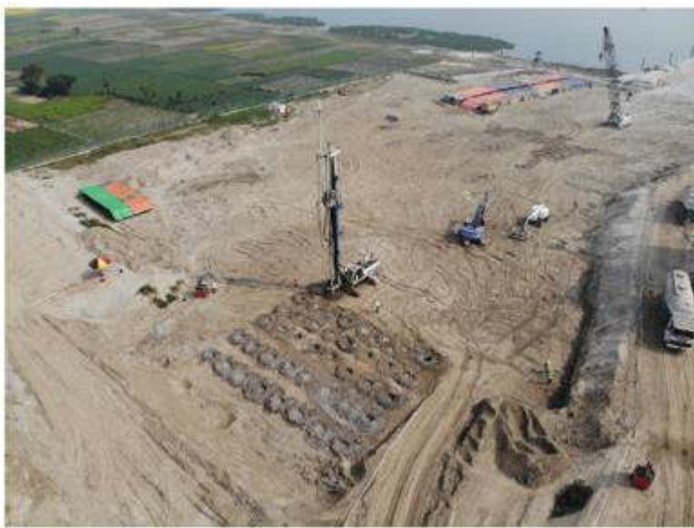
Photo A.2: DSM construction at intake Site, 19 January 2020
