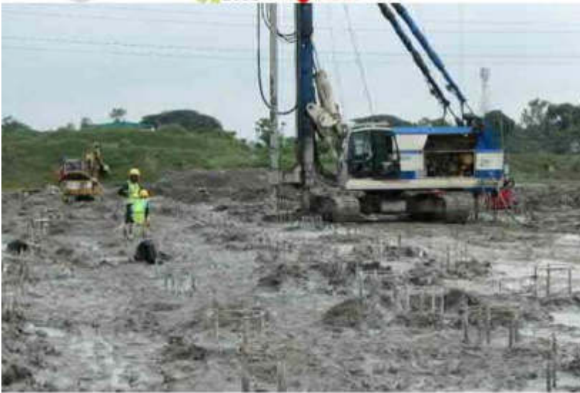
Photo A.4: DSM construction at WTP Site, 14 June 2020
