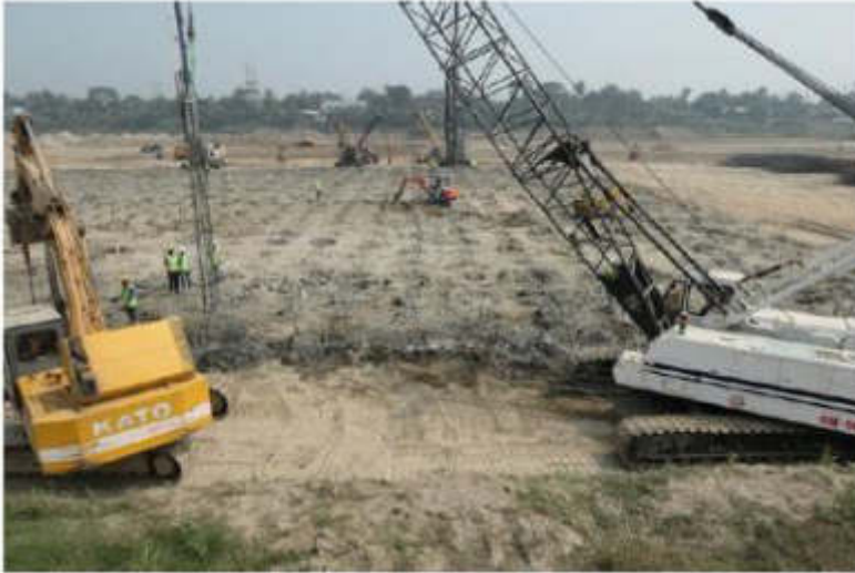
Photo A.4: DSM construction at WTP Site, 14 June 2020
