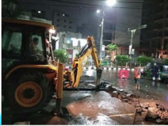
Road breaking for interconnection at DMA64
