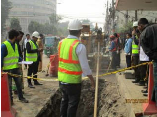
200 mm dia HDD running at DIT ave. DMA 615, Neapali team are in visit
