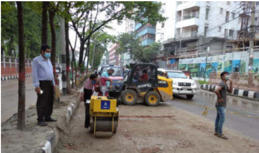
Rd Filling & compaction: Shahjahanpur DMA615, SARE MSC at site on 13.06.20
