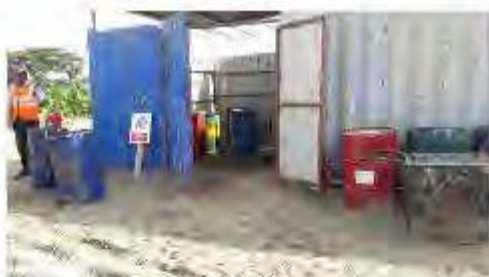
Fuel storage is poor
