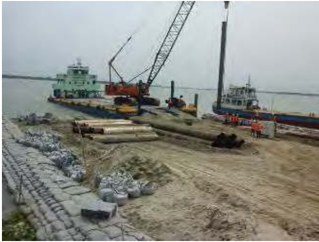
Photo A.1: Jetty construction at intake Site, 25 September 2019
