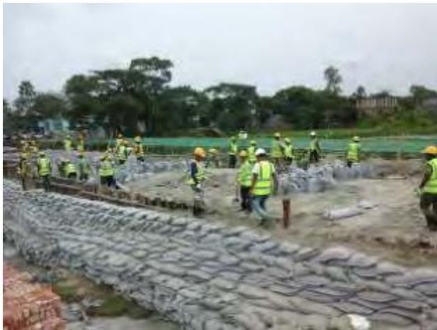
Photo A.2: Temporary road construction at intake Site, 25 September 2019
