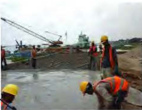
On going Jetty construction at River Side
