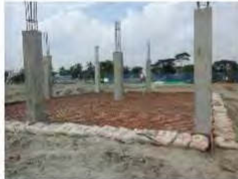
Ongoing reinf. placement in temporary works
