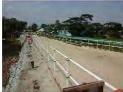
Temporary access road construction completed
