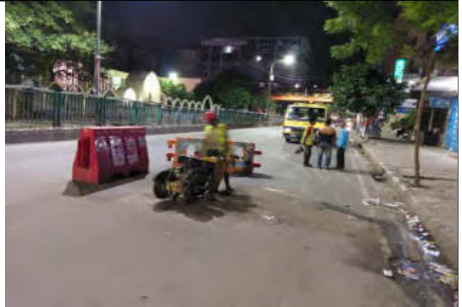
Road cutting by cutter machine at Purana Paltan DMA 615 on 02.09.18
