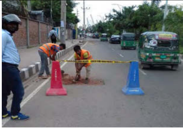
HDD pit cutting at DMA 610 Hatir Jheel road
