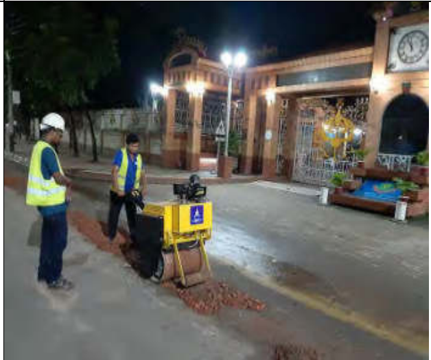
Road compaction and rolling In front of police HQ
