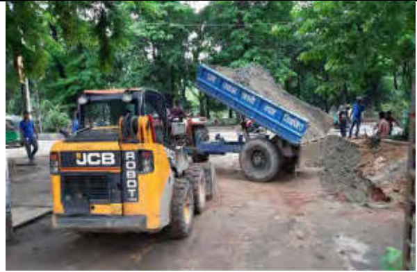
Back filling at DMA 614, Minto road on.8.07.19
