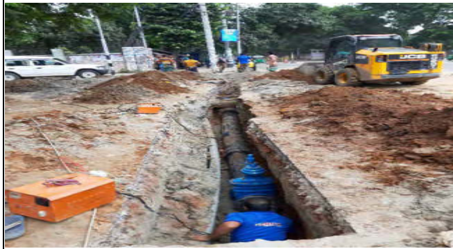
HDD pit cutting at DMA 610 Hatir Jheel road
