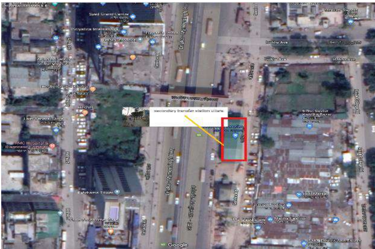
Photograph of Secondary Transfer station, Uttara.
