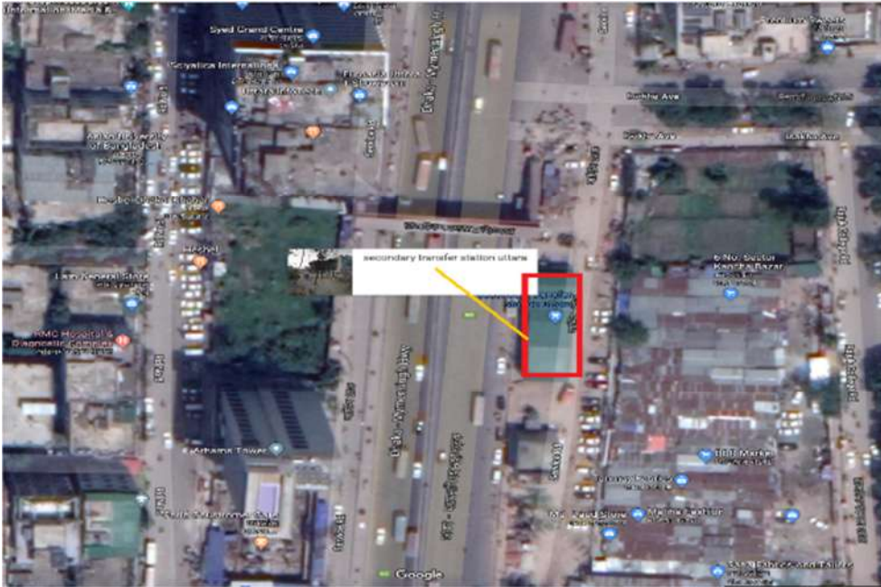
Photograph of Secondary Transfer station, Uttara.
